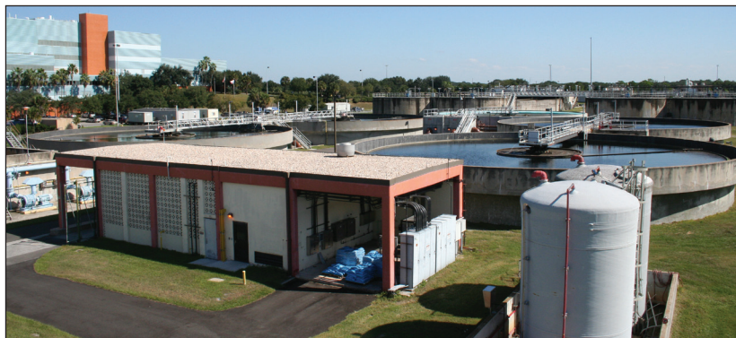
The Falkenburg Wastewater Treatment Plant in Brandon receives electricity directly from the County's Resource Recovery Facility next door, saving thousands of dollars each month.
